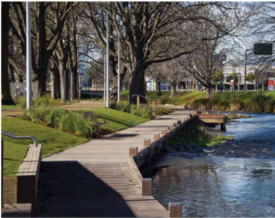
Watermark demonstrates the use of boardwalks and landscaping to enhance the look of the riverbanks, and works to restore river ecology.
