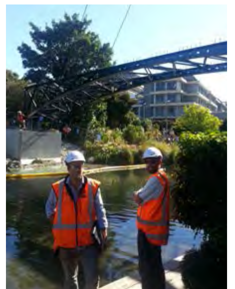
Downer project manager Alex Mowe and bridge designer Campbell Apthorp watched from the sidelines as the Antigua Street footbridge was lowered back into place last month.
