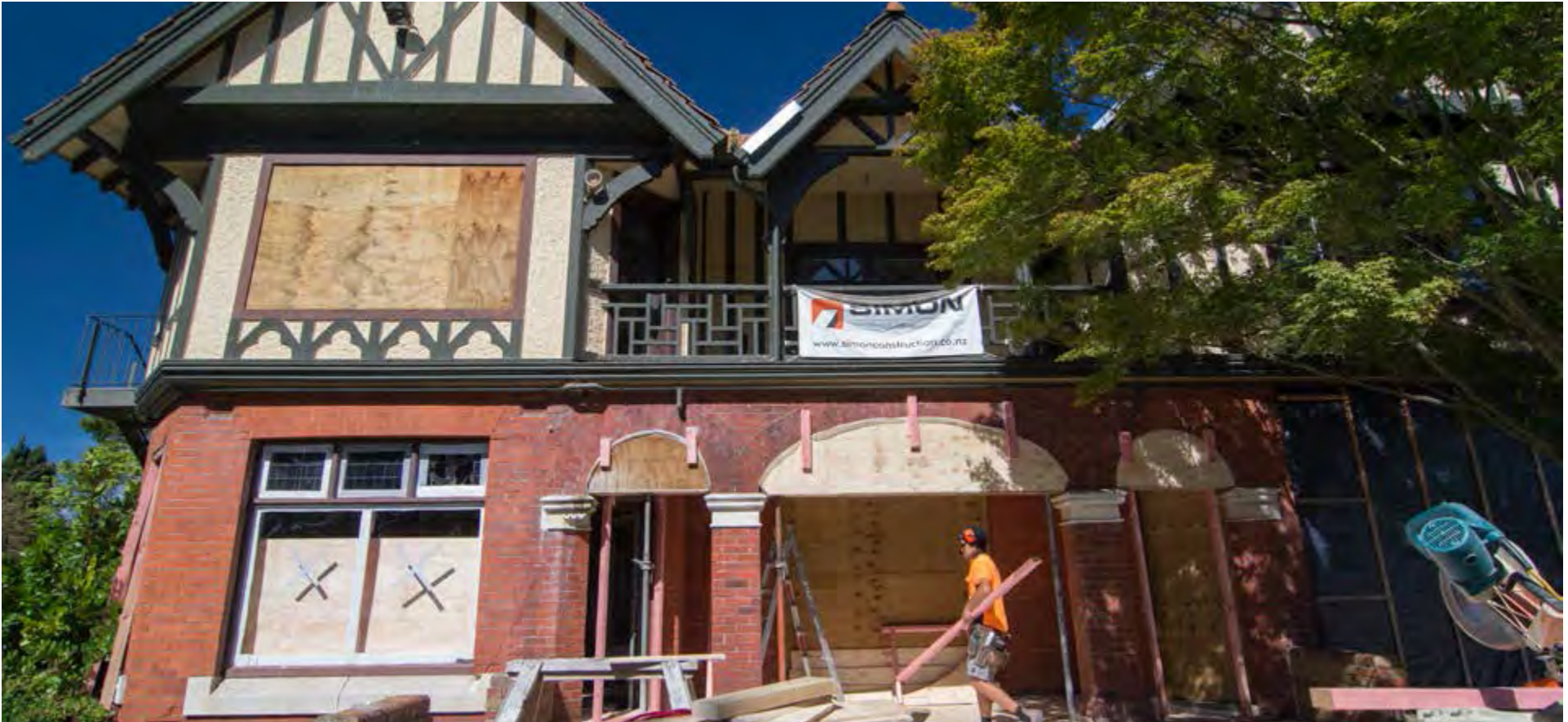
Restoring a Christchurch treasure: Work underway on the Mona Vale Homestead.
