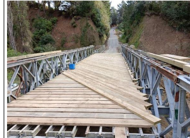
Construction of the Follies Bailey bridge is progressing well.
