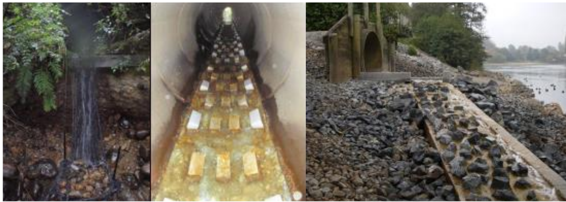
Figure 12: Examples of techniques to retrofit fish migration barriers. Left: oyster spat ropes for climbing galaxiids (photo Bruno David, Waikato Regional Council). Middle: culvert flow baffles. Right: rock ramps (photos Paul Franklin, ©NIWA).
