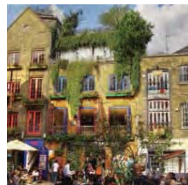
Shops and residences at upper levels contribute to texture, activity and surveillance.
