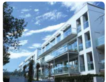
Madison Apartments, Christchurch
