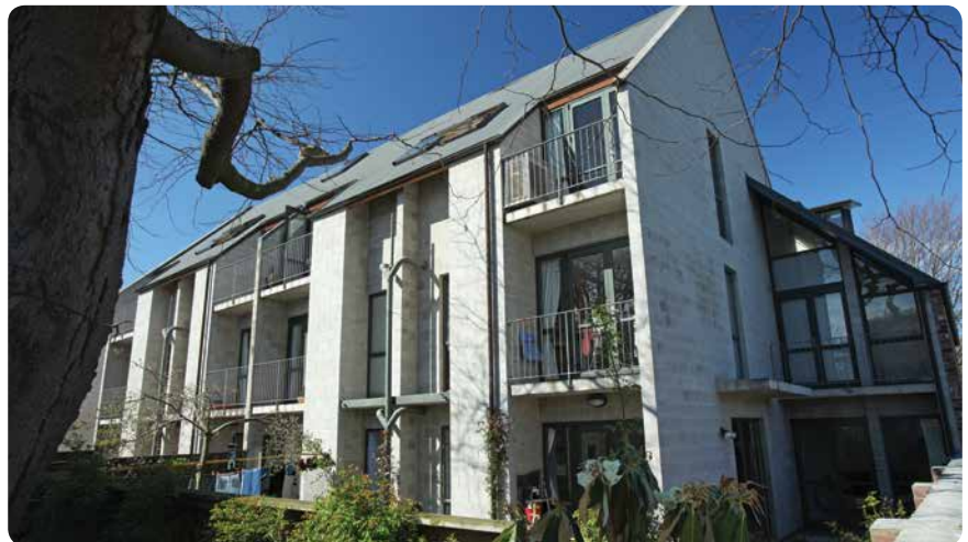
St Mary's Apartments, Christchurch
