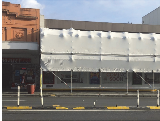
Figure 16 Example of building shrink wrap on a building worksite on Karangahape road
